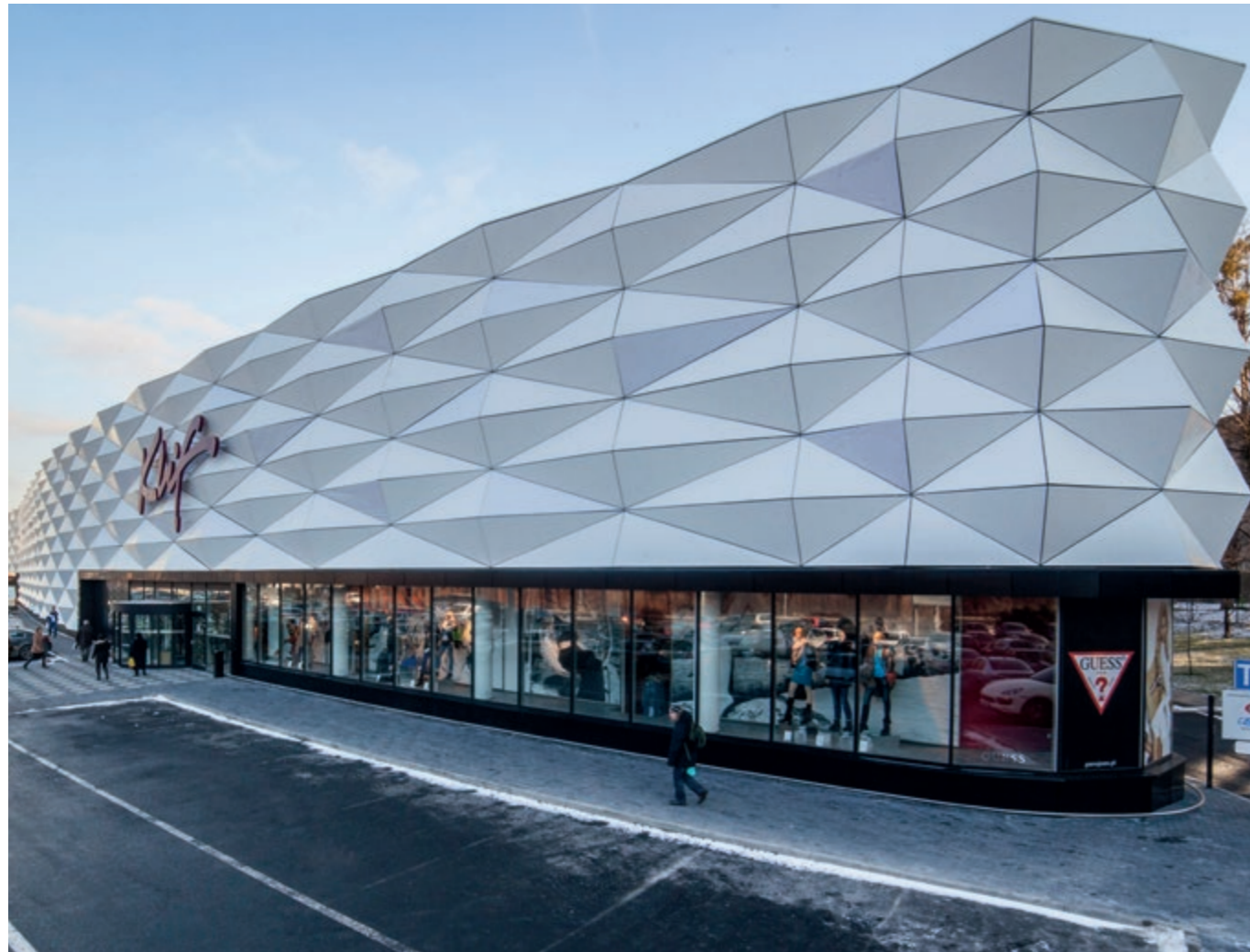
ABOVE: Corian® Exteriors panels made from Corian® Solid Surface Glacier White for the facade of the Dom Mody Klif shopping mall in Warsaw, Poland; Warszawa"; project Architect: Grupa 5 (investor: PAIGE Investments); photo by Corian® Exteriors, all rights reserved. OPPOSITE: The Microsoft Germany headquarters in Munich. The building's exterior is enveloped with Corian® Exteriors panels (made from Corian® Solid Surface Glacier White) which feature a fascinating depth when illuminated by the sun. Project by GSP Architekten Munich; facade by HAGA Metallbau GmbH; photo by Andreas Frisch, GSP Architekten, all rights reserved.
