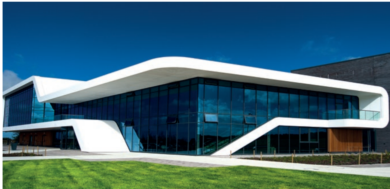
ABOVE: Corian® Exteriors panels (made with Corian® Solid Surface Glacier White) for the facade of Menai Science Park in Gaerwen, Wales; project by FaulknerBrowns Architects; photo courtesy of CD (UK) Ltd., all rights reserved.
